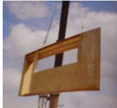
Slika 40: Prefabricirana stena (Vir 1)
